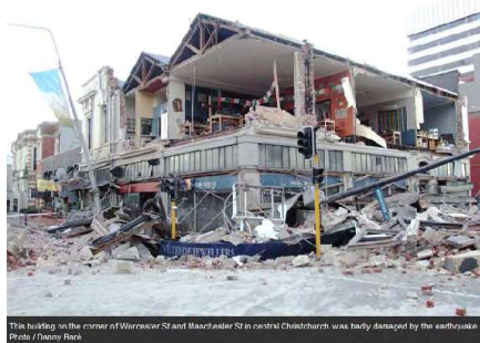
This building on the corner of Worcester St and Manchester St in central Christchurch was badly damaged by the earthquake. Photo / Henry Raze
