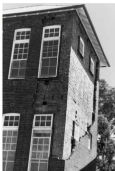
▲ 11.4 Damage to brick veneer due to corroded veneer ties. 1969 Newcastle, Australia earthquake. (Reproduced with permission from R.B. Sheehar).
